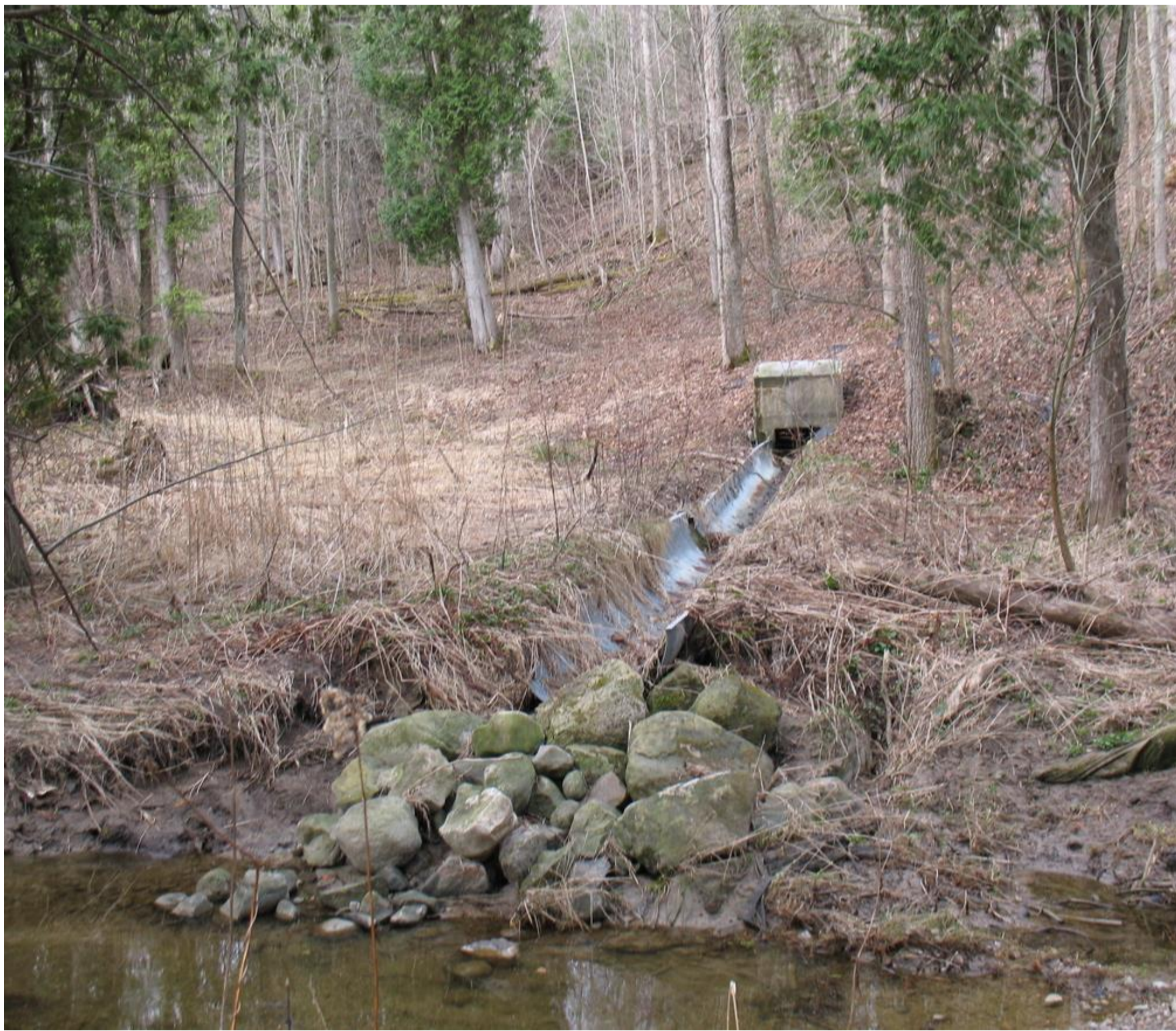
Outfall discharge at side channel
