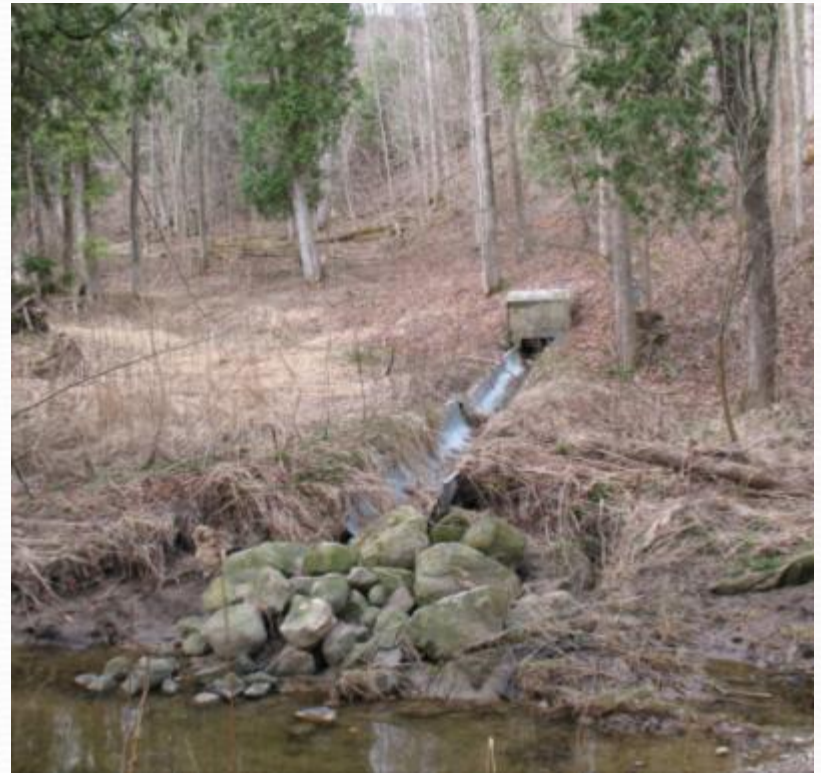
STP Outfall at River
