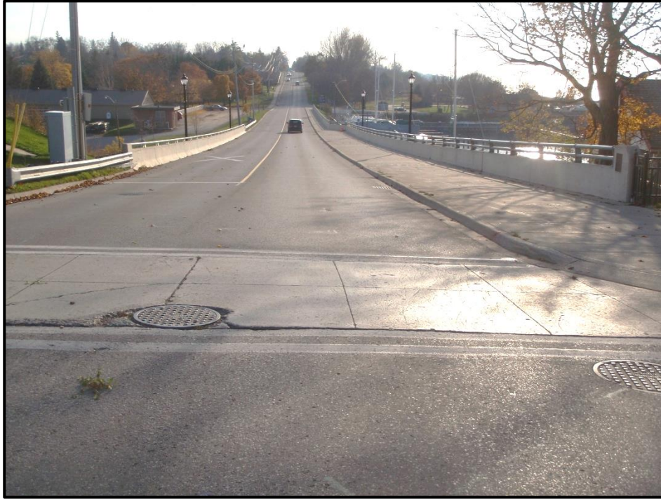
Image 3: Overview of Bridge on Huron Terrace across Pentagore River (looking south)
