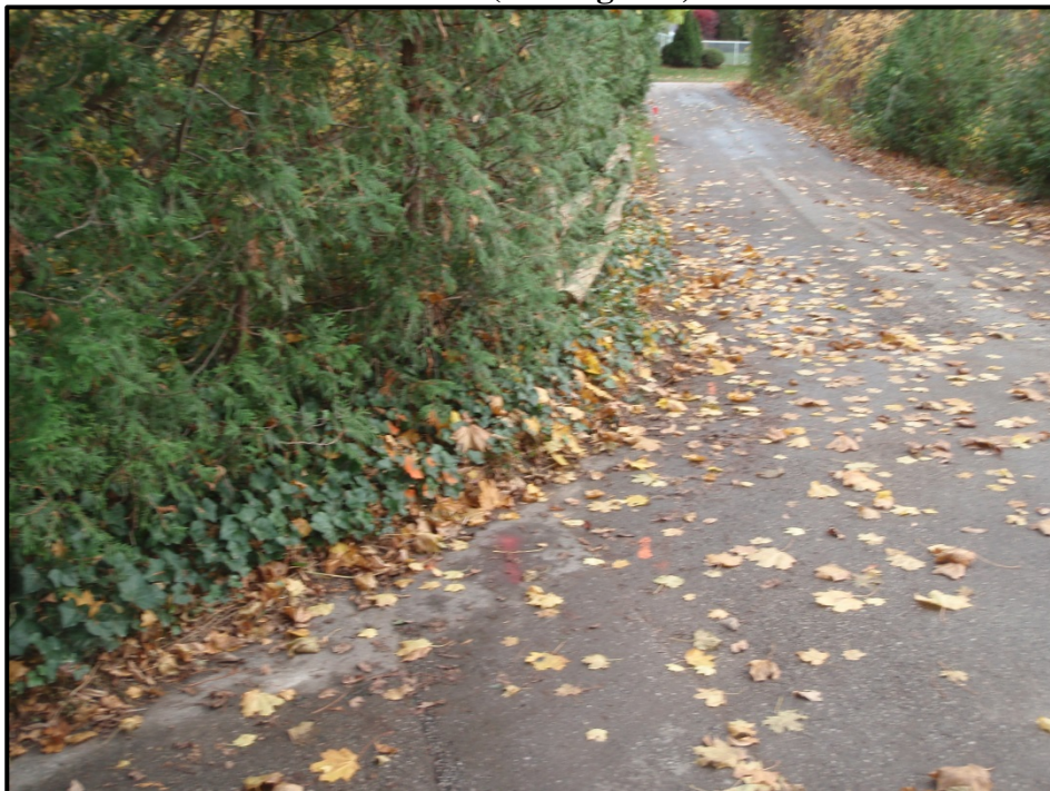
Image 27: Existing Conditions on Paved Laneway to Golf Course Pathway (looking north)
