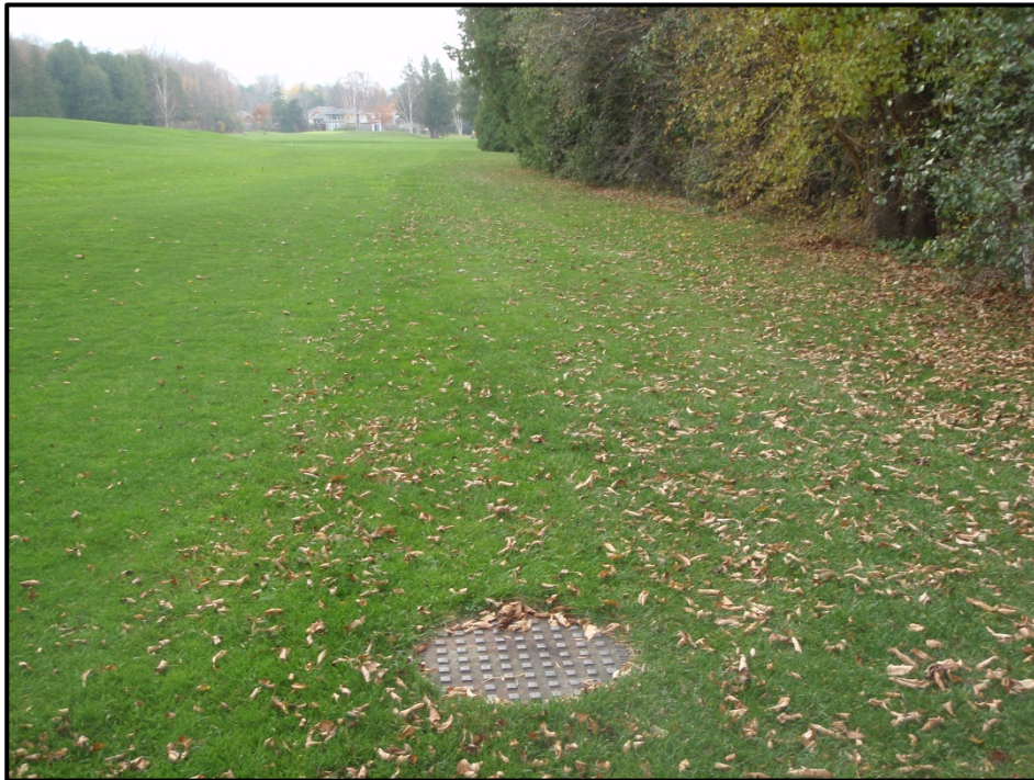
Image 31: Termination of Sanitary Line Improvements at Golf Links Road (looking south)
