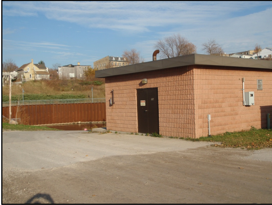
Image 1: Huron Terrace Sewage Pumping Station (SPS), on South Side of Pentagore River (looking northeast)
