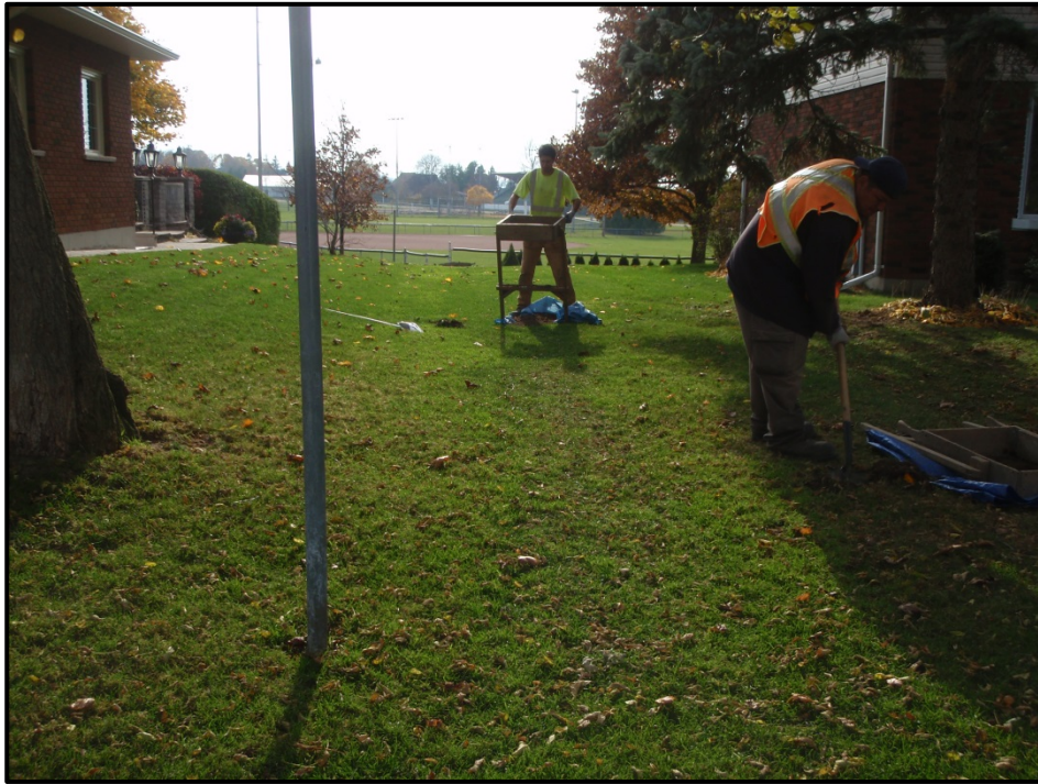
Image 22: Course of Pipe on Kingsway Street (looking west)
