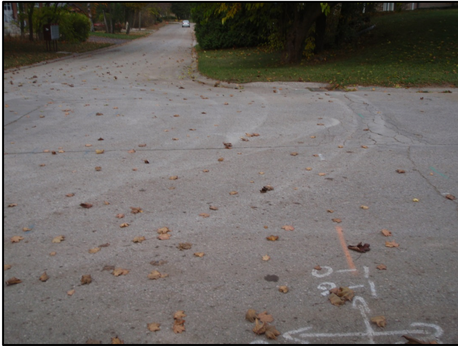
Image 24: Existing Conditions along Corridor on Shevchenko Boulevard (looking south)
