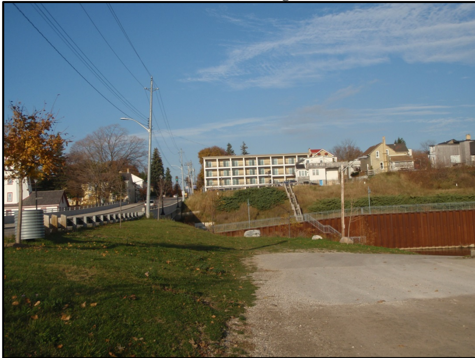
Image 2: Existing Conditions on South and North Side of Pentagore River at Huron Terrace SPS (looking north)
