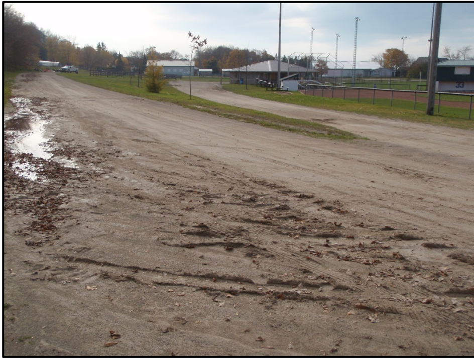
Image 18: Overview of Grassed Area between Track and Parking Area (looking north)
