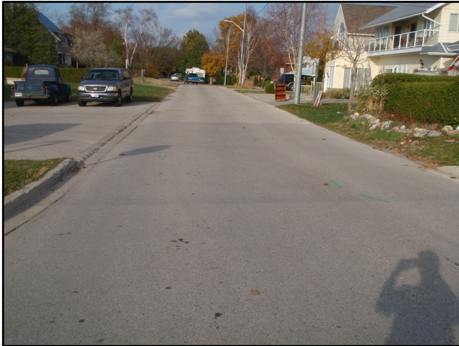
Image 10: Saugeen Street, South of Broadway (looking south)
