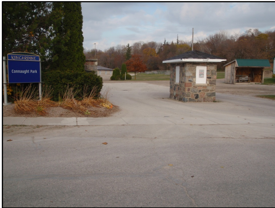
Image 14: Course of the New Force Main and Sanitary Line from Park Entrance (looking southwest)
