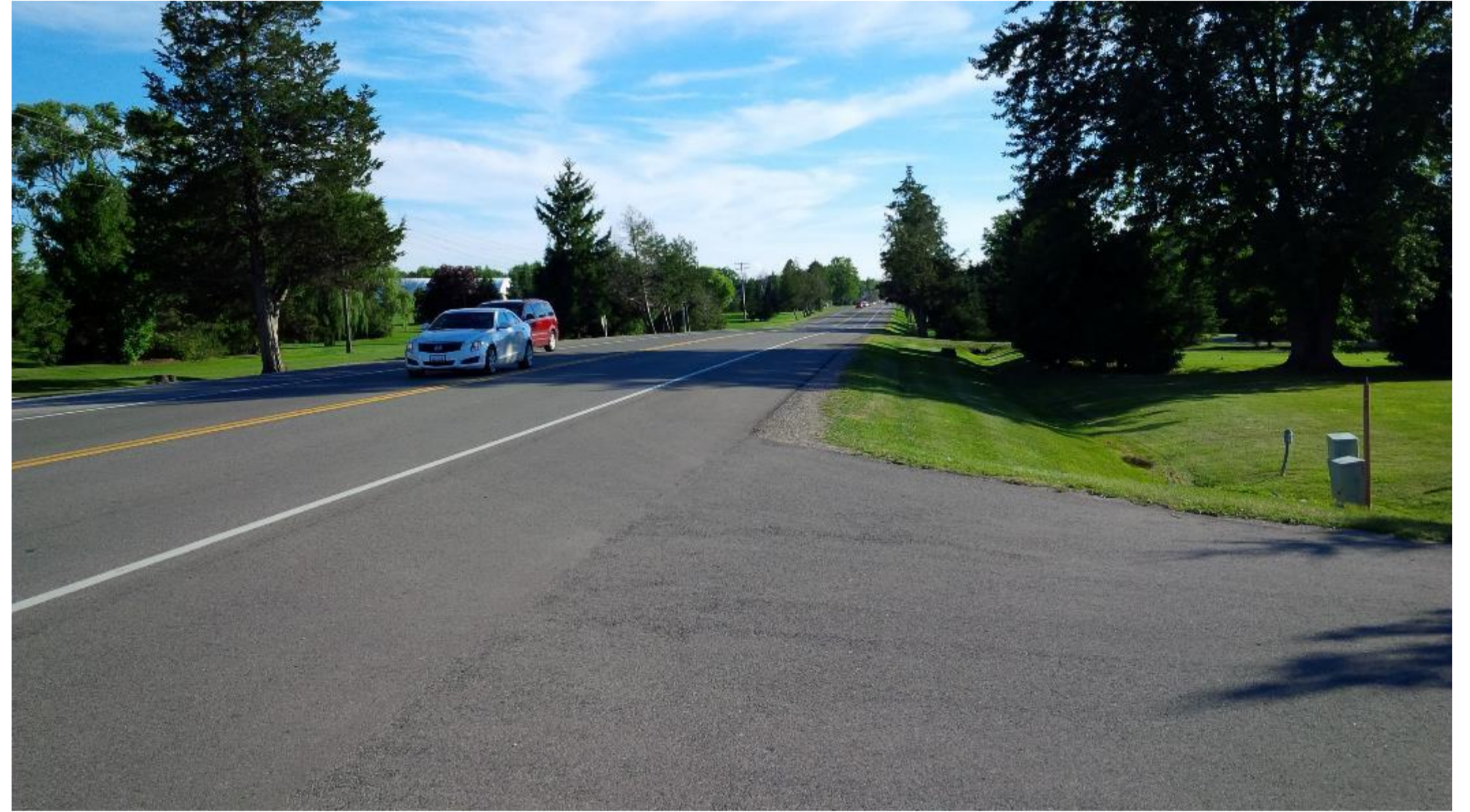
Corridor adjacent to Oakwood
