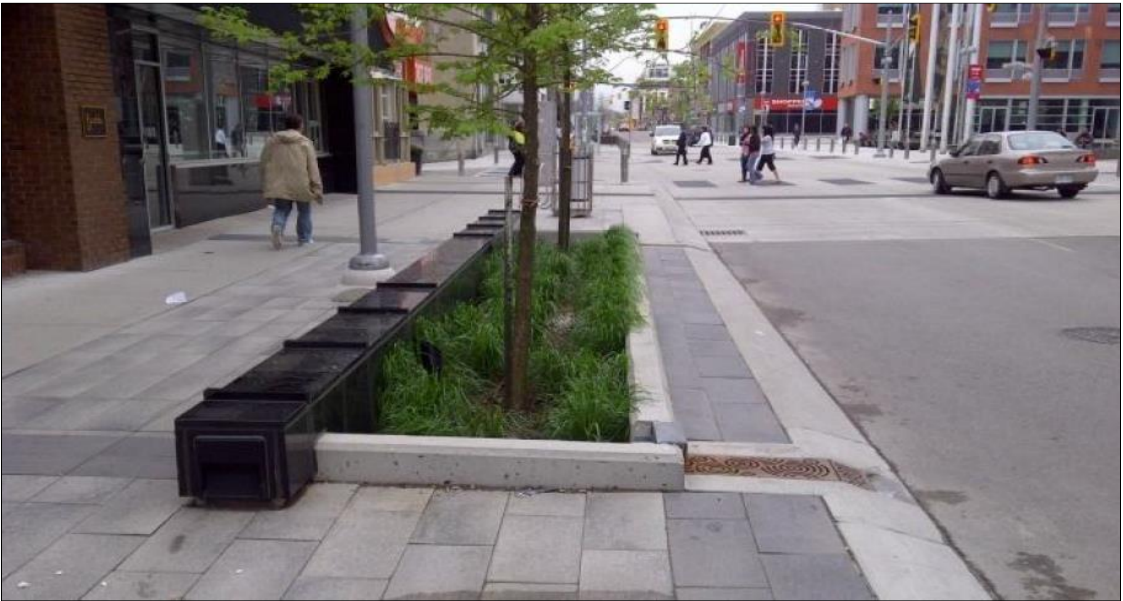
Bioretention Boulevard Planters, King Street – Kitchener
