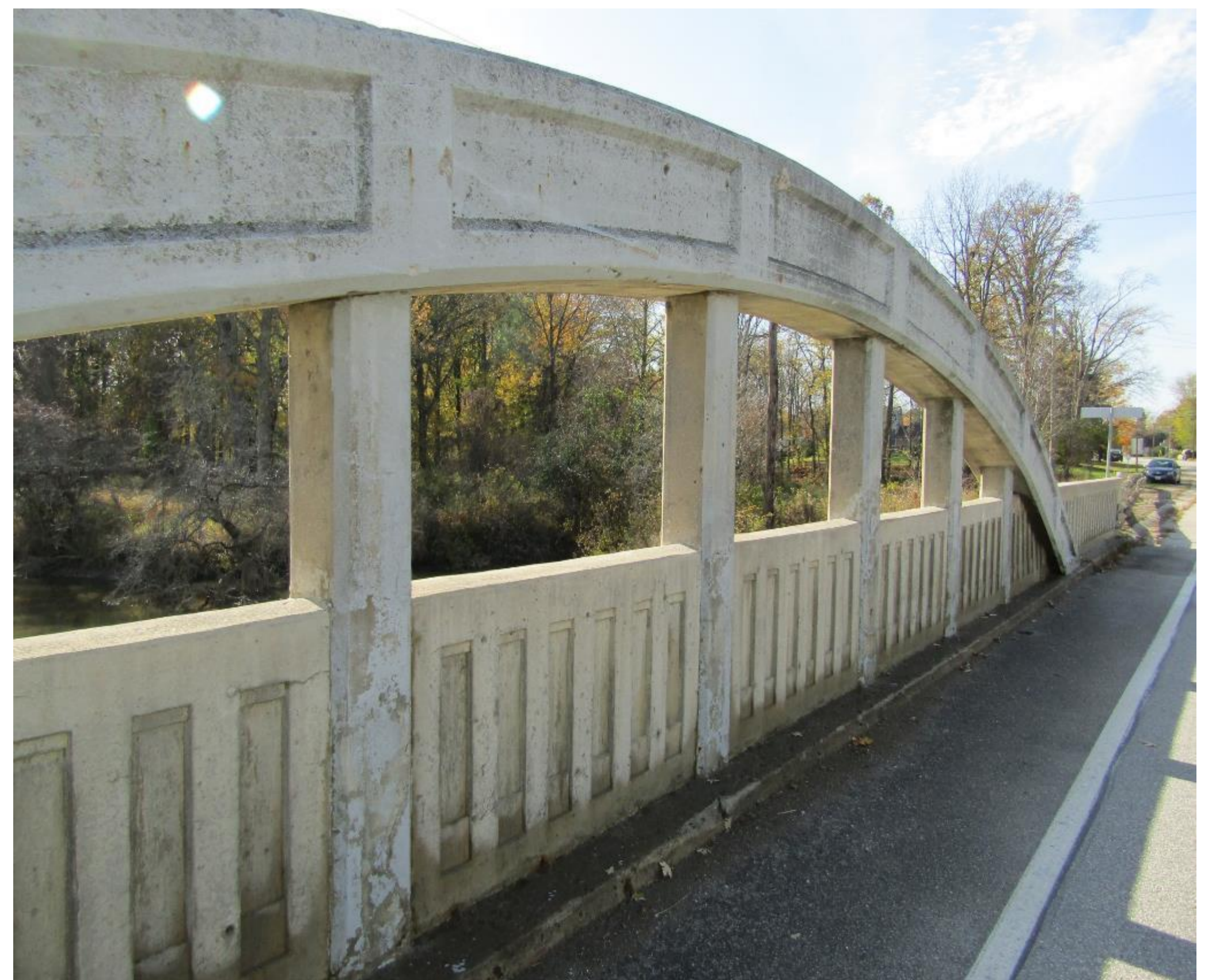
VIEW SHOWING CONCRETE PANELING SET INTO ARCHES
