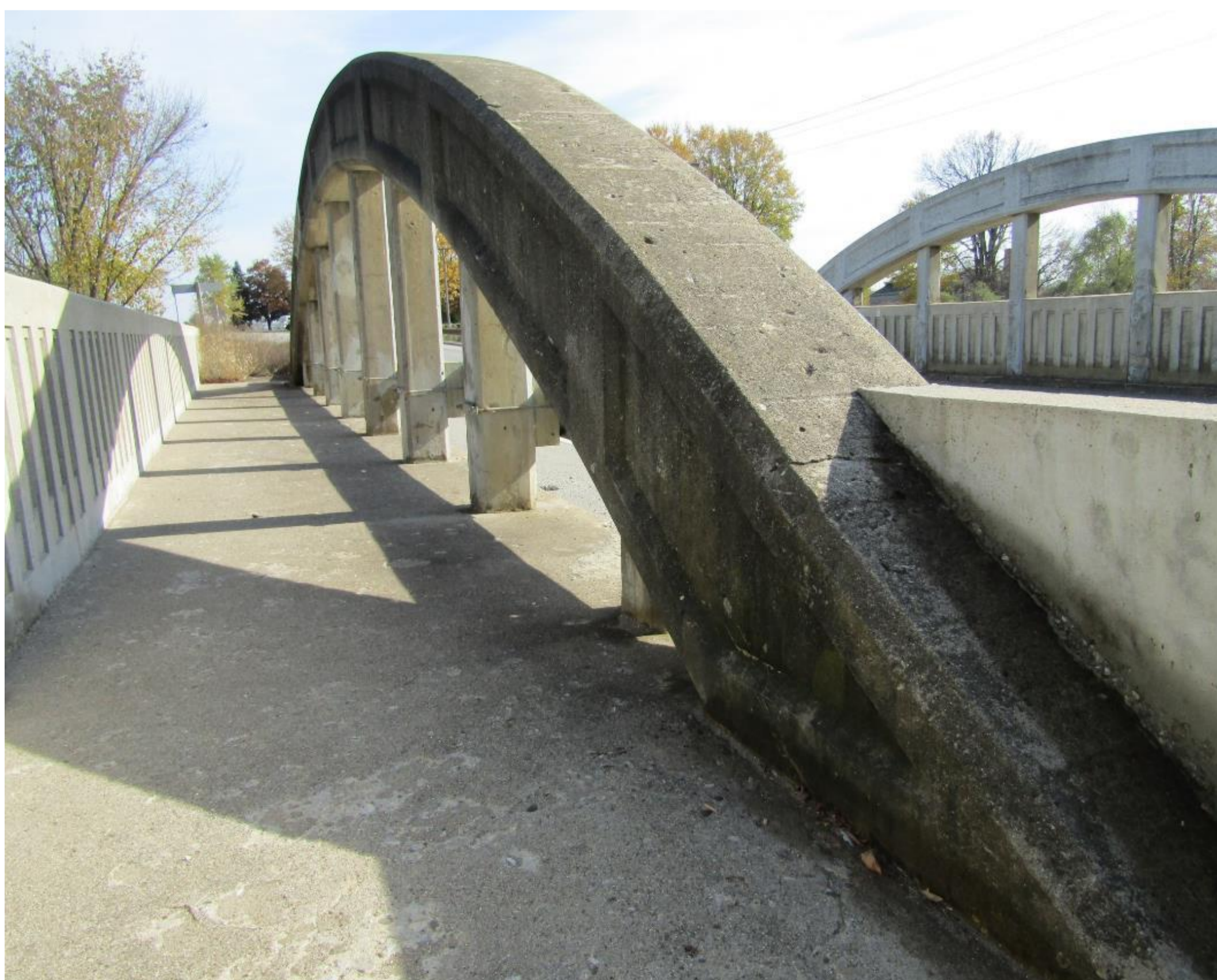
VIEW SHOWING SYMMETRICAL ARCHES AND CONCRETE SIDEWALK
