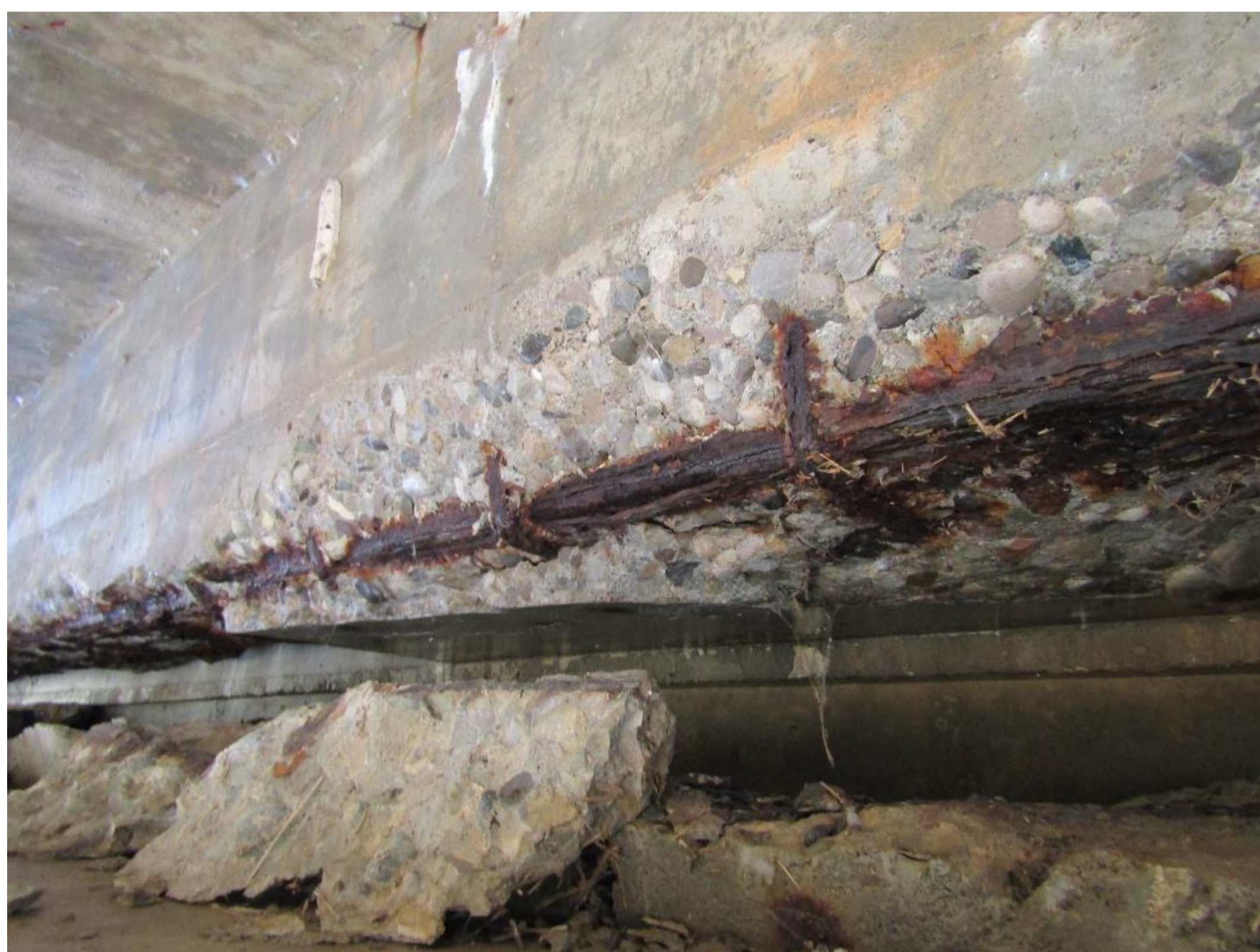
EXPOSED REBAR
