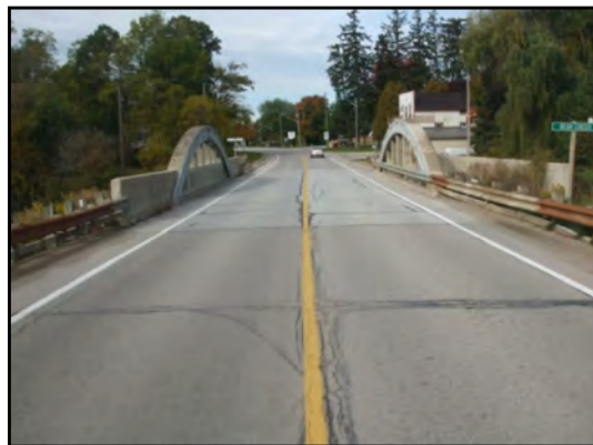
EGREMONT ROAD FACING WEST
