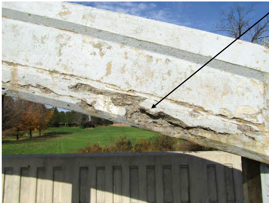
Arches in poor condition
