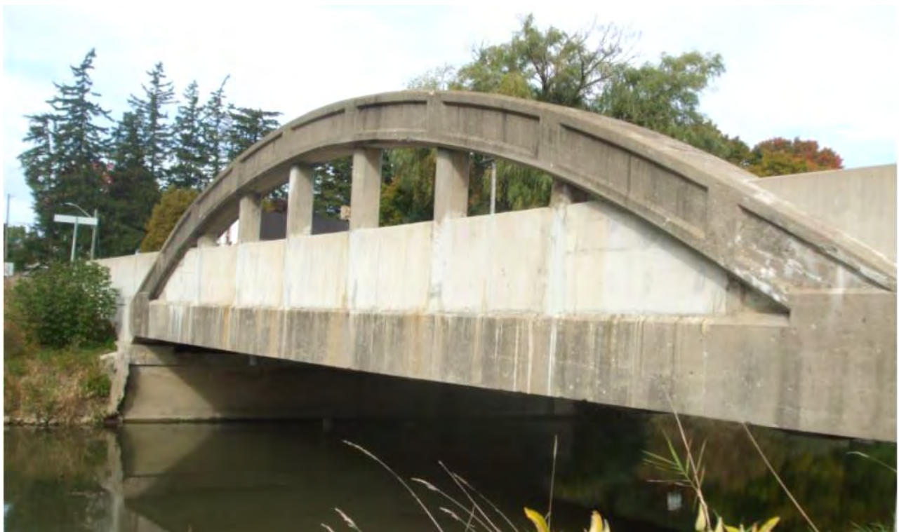
▲ Photo of the Bear Creek Bridge south elevation
