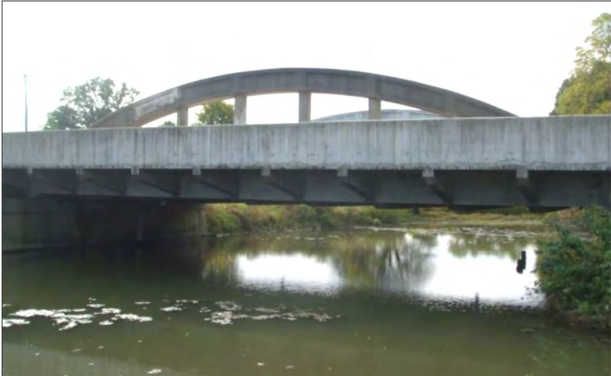
Photo looking south toward the existing bridge and stream channel ↑
