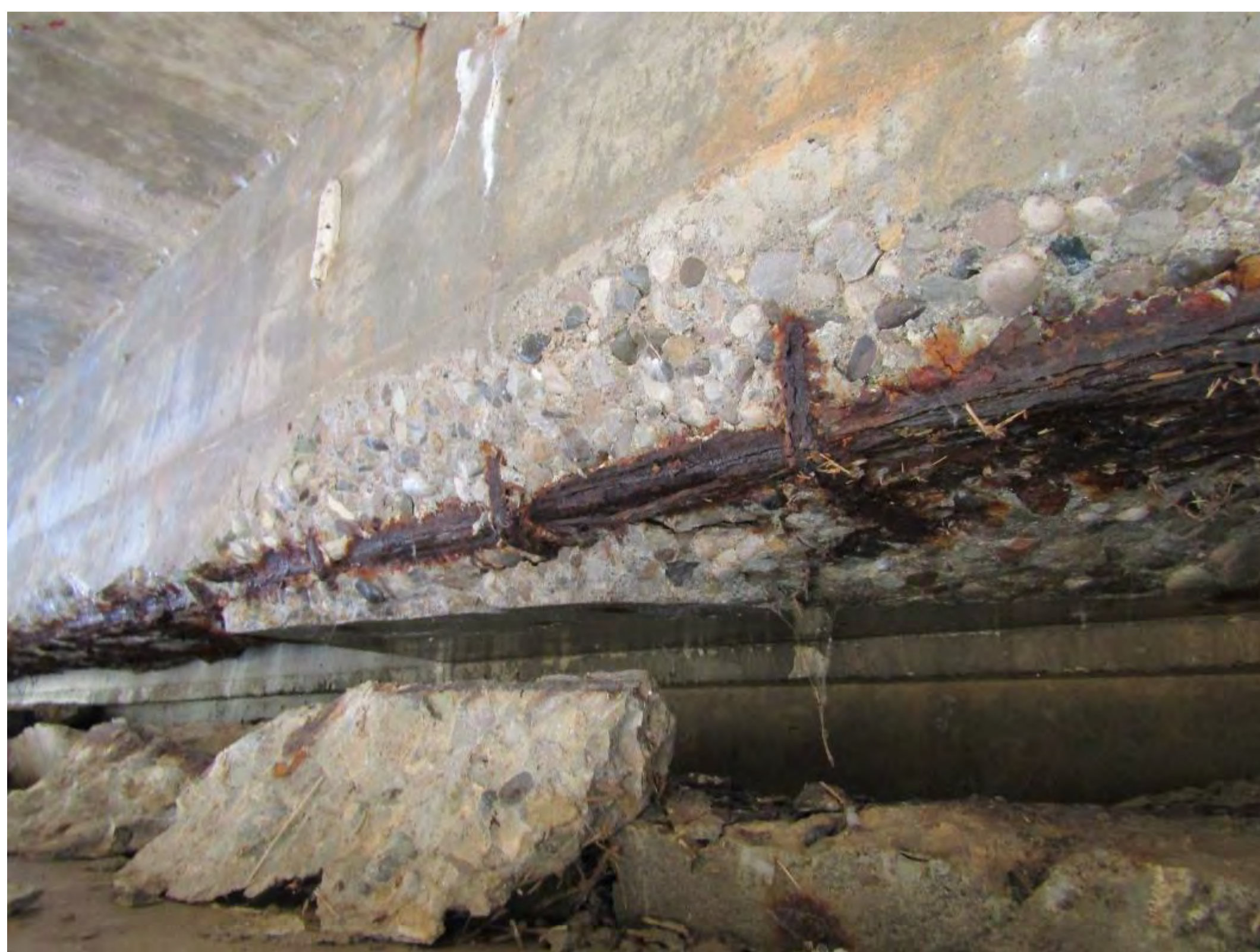
EXPOSED REBAR
