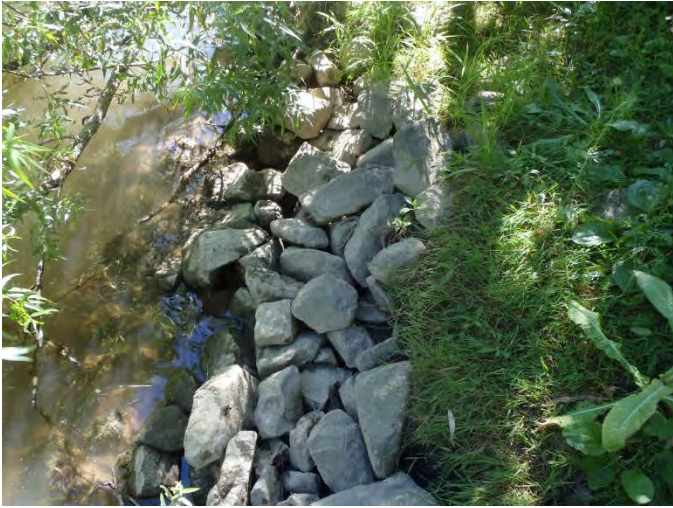
Photo 8: Rip rap along bank of Bear Creek channel
