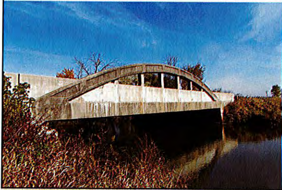
SOUTH SIDE OF BRIDGE
