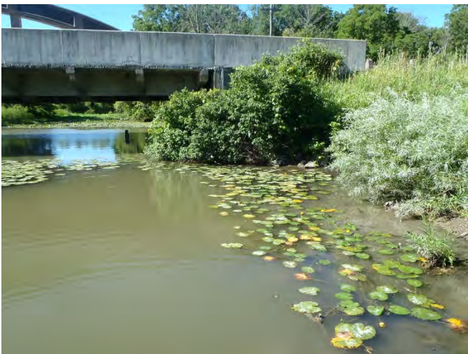
Photo 2: Upstream side facing south towards bridge (west side)
