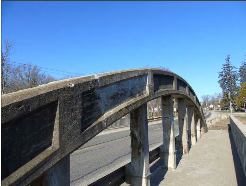
Image 18: Detail showing concrete panelling of concrete arch
