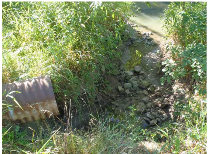
Photo 15: Culvert to the west of bridge
