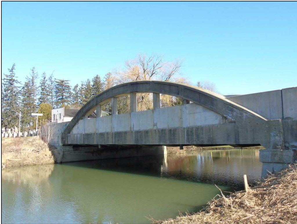
Image 24: View showing south side of the bridge showing un-textured concrete
