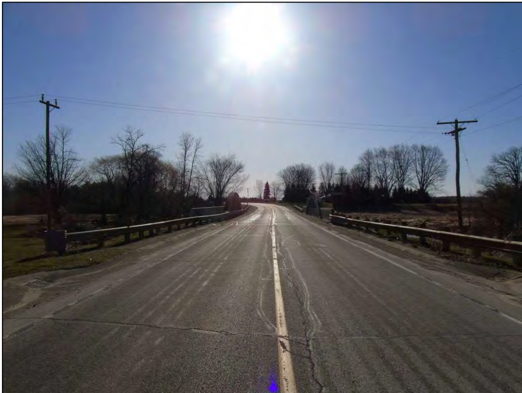
Image 10: View looking east towards Bear Creek Bridge
