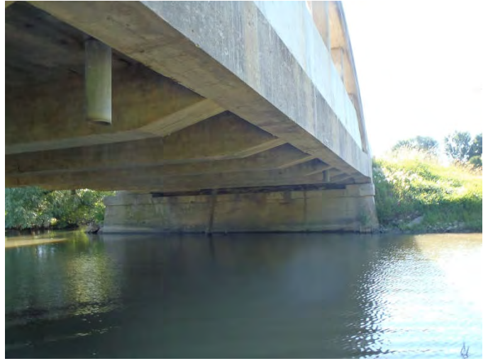
Photo 14: Bridge (downstream side facing east)
