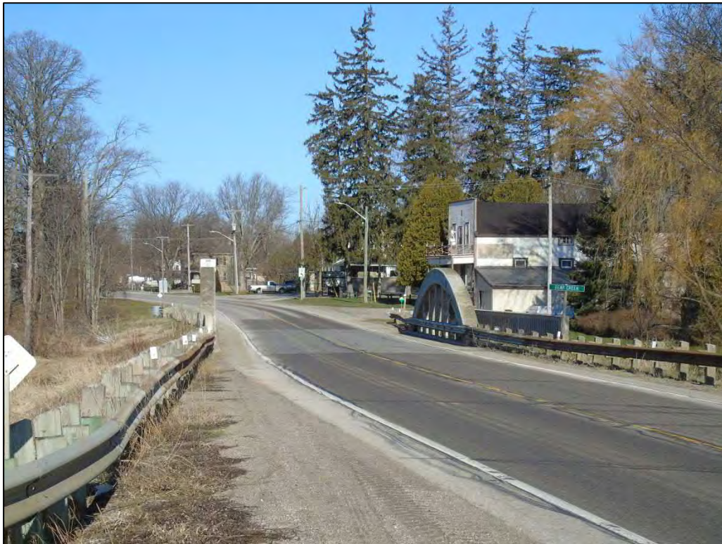
Image 12: View looking west, showing Bear Creek Bridge and Warwick village in background
