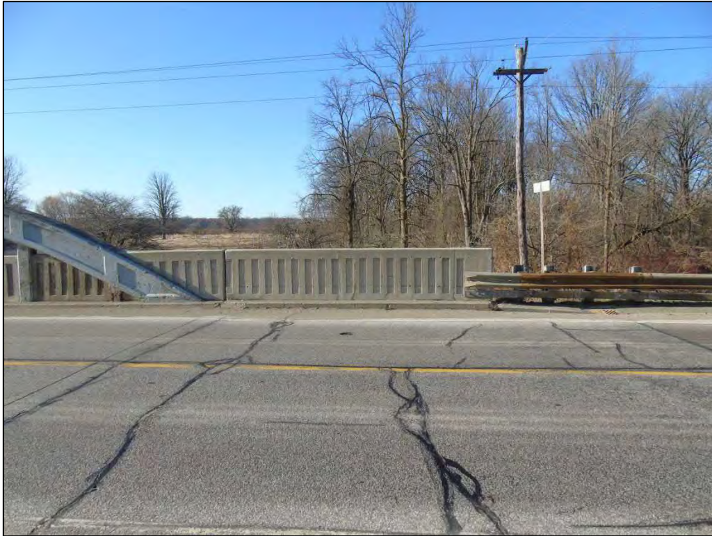
Image 22: View showing concrete guardrail on the south side of the bridge
