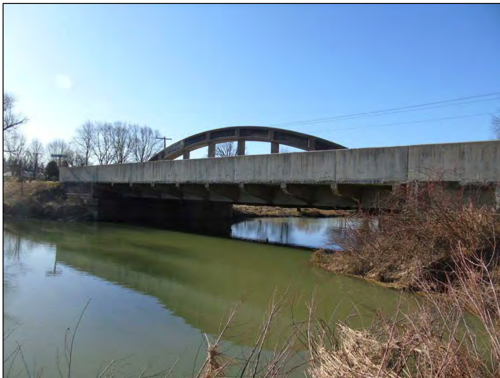
Image 25: View showing north side of the bridge
