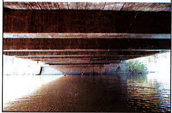
UNDERSIDE OF BRIDGE FACING EAST
