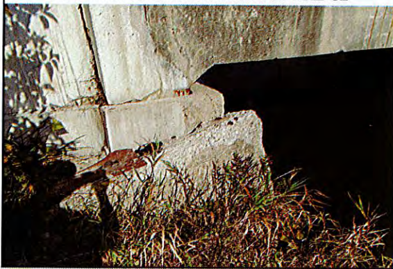
ABUTMENTS ON NORTH SIDE OF BRIDGE
