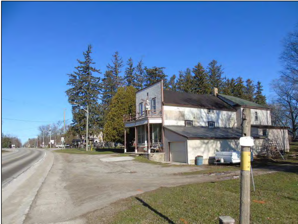
Image 9: Warwick General Store, located immediately west of the bridge
