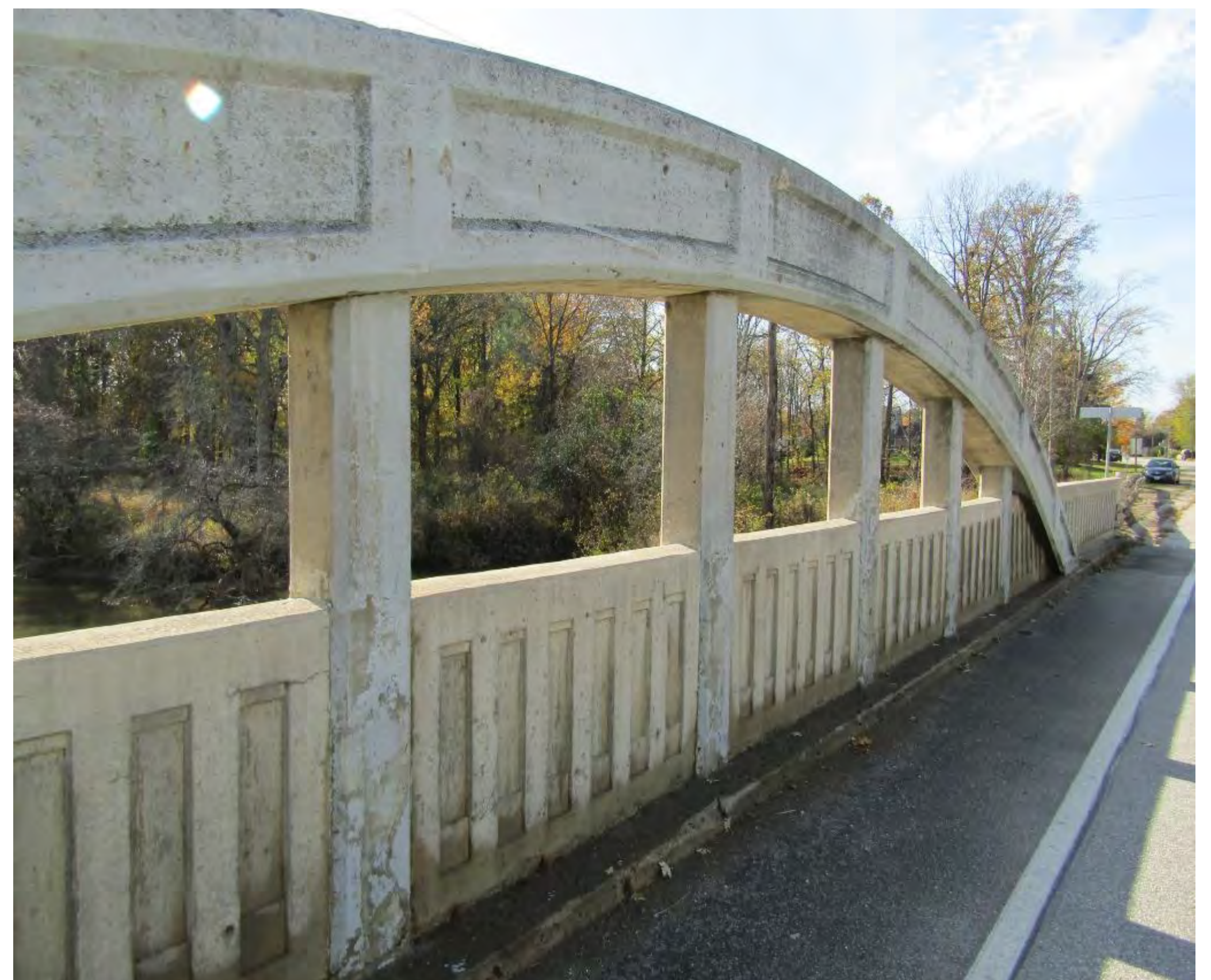
VIEW SHOWING CONCRETE PANELING SET INTO ARCHES
