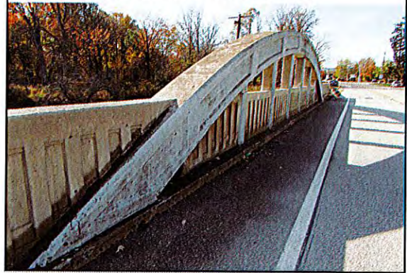
VIEW SHOWING SOUTH ARCH
