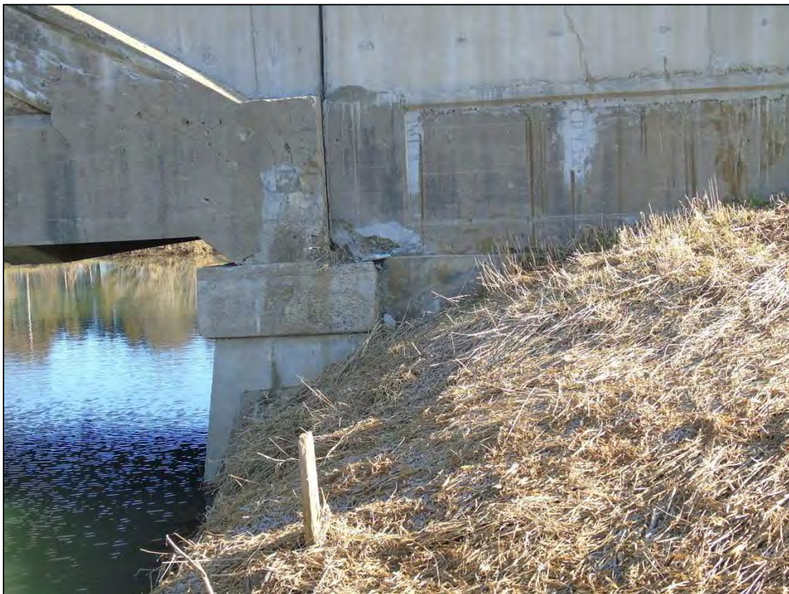
Image 15: Detail showing concrete west abutment of Bear Creek Bridge
