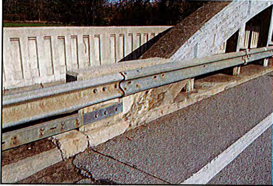
GUARDRAIL ON NORTH SIDE OF BRIDGE
