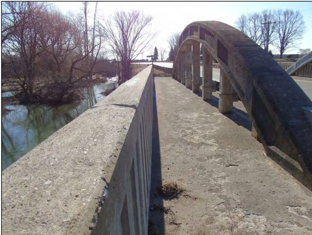
Image 20: Detail showing concrete guardrail and concrete sidewalk on north side of the bridge
