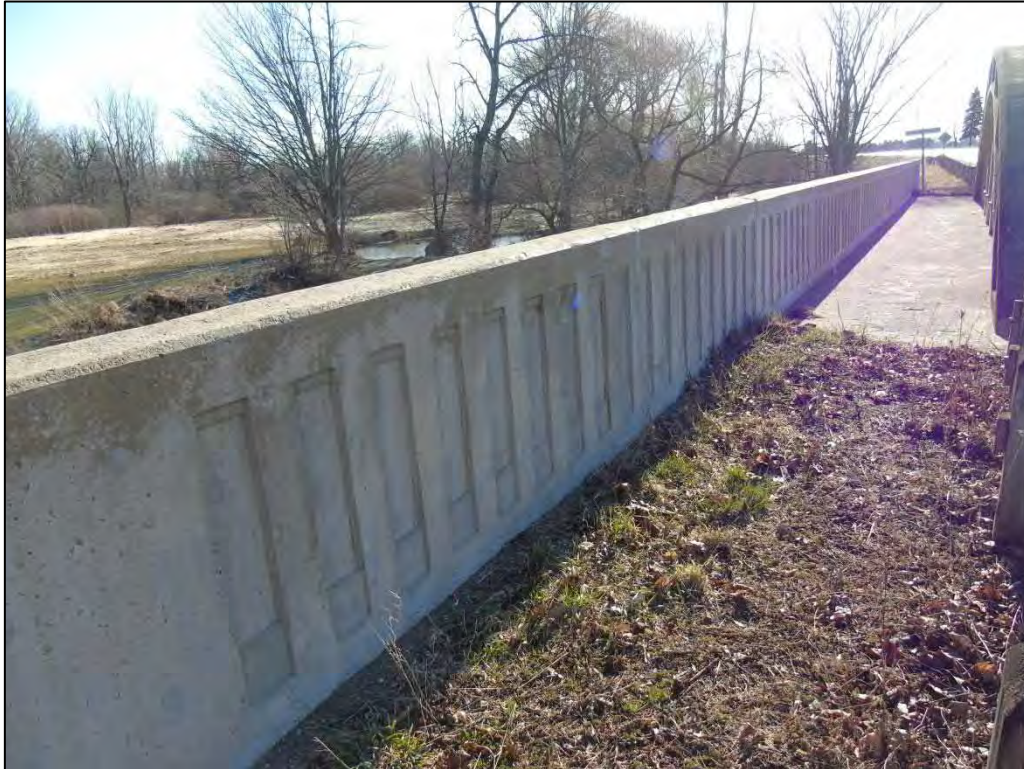
Image 21: Detail of concrete guardrail on north side of the bridge
