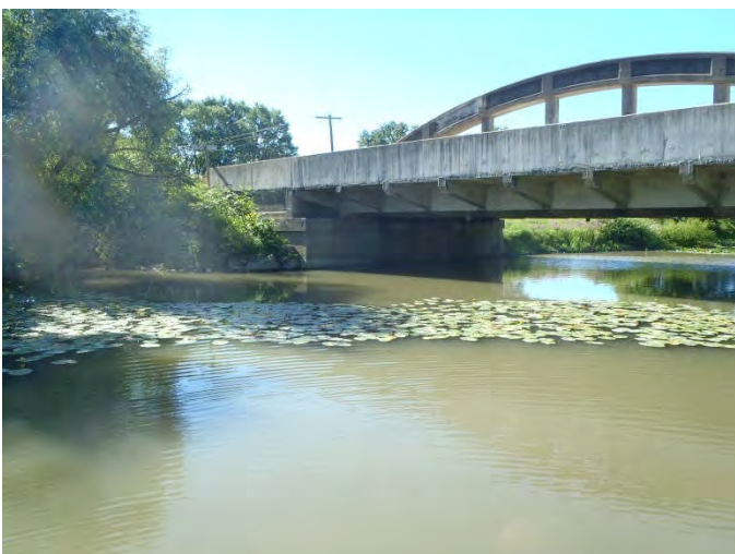
Photo 3: Upstream side facing south towards bridge (east side)
