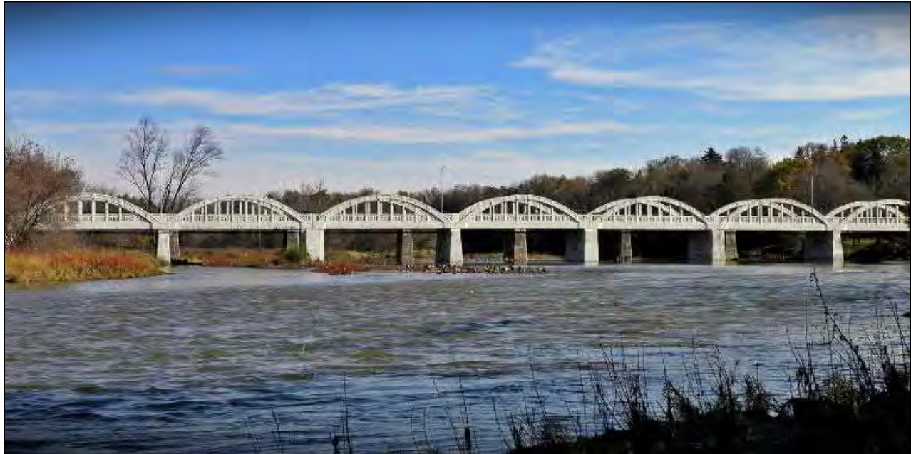
Image 14: Freeport Bridge, Kitchener, Ontario, showing one of the most well-known concrete bowstring arch in southern Ontario (Google Images, 2018)
