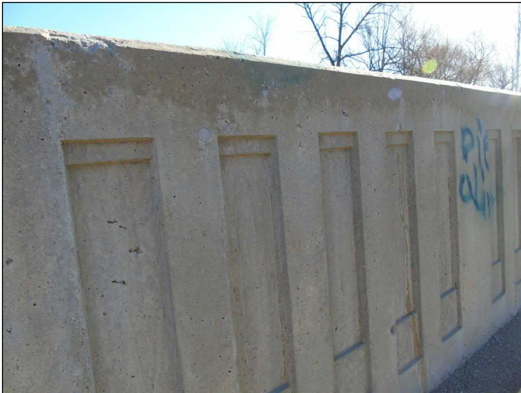
Image 23: Detail of concrete panelling on guardrail
