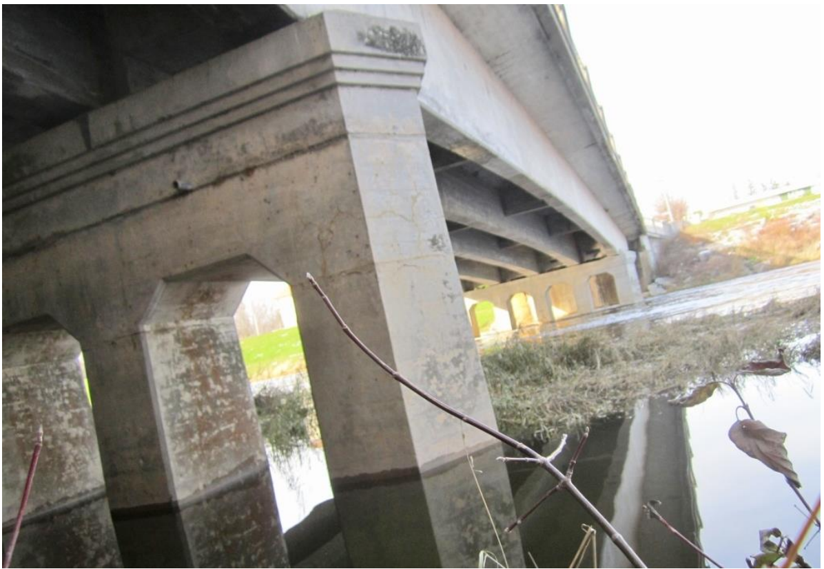
View of the south pier
