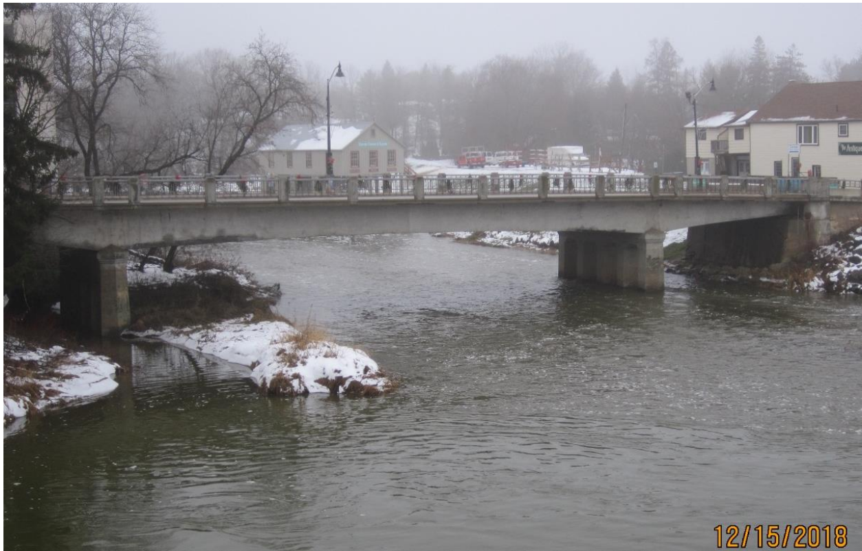
View of east elevation of Bridge
