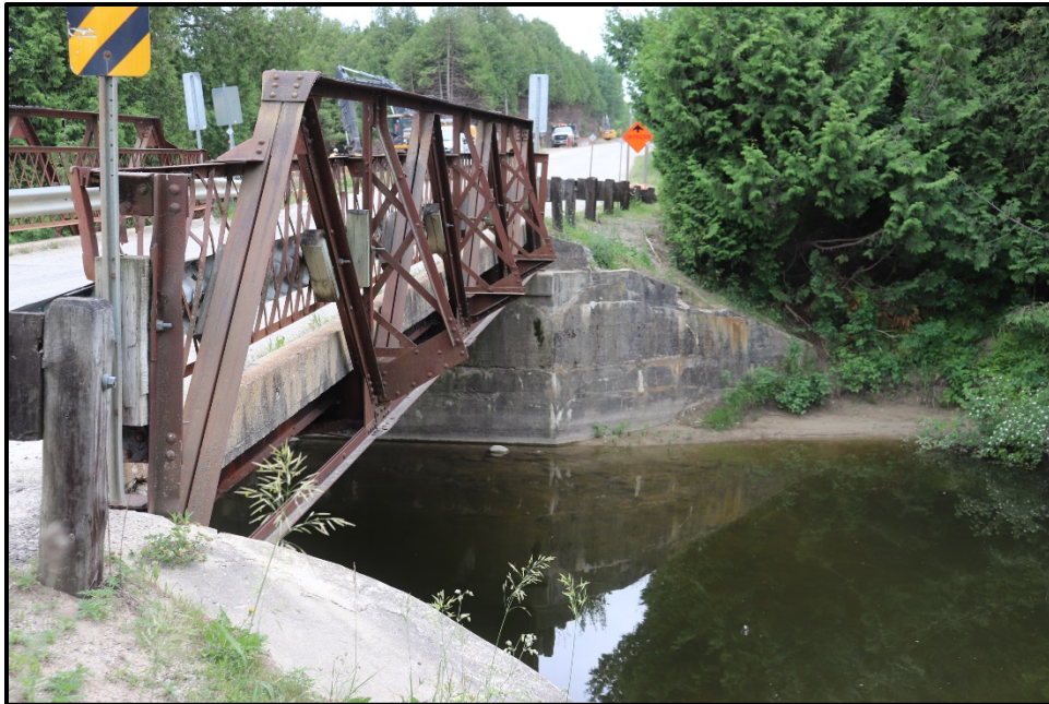
Image 5: West side truss structure with outriggers and south abutment (TMHC 2020)
