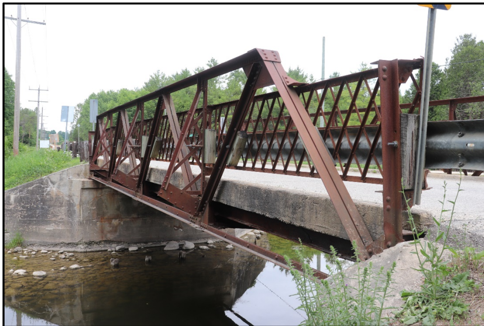
Image 1: East side and south abutment of Lantz Bridge (TMHC 2020)
