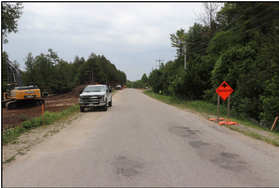
Image 11: View south from bridge showing rural landscape and construction activities (TMHC 2020)
