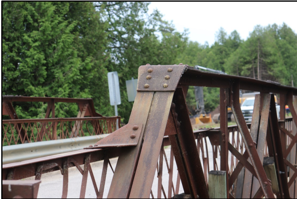
Image 8: Detail of riveted truss construction (TMHC 2020)
