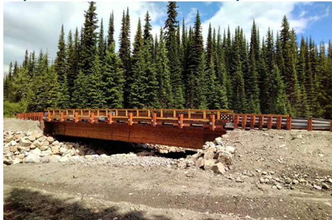
22m Clear span bridge with wood superstructure bridge
