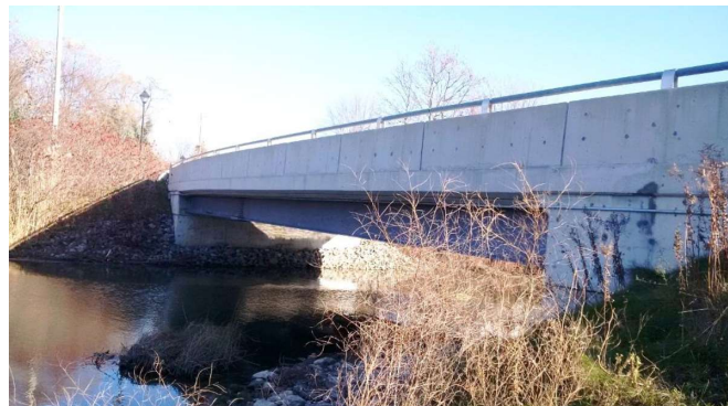
24m span steel girder with concrete deck and barrier walls
