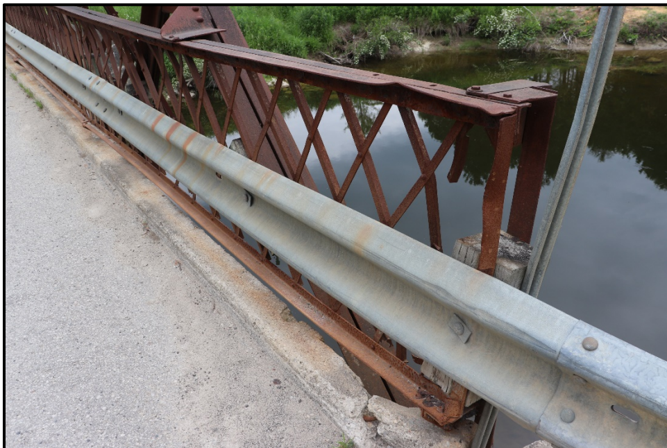
Image 9: Detail of lattice style handrail (TMHC 2020)
