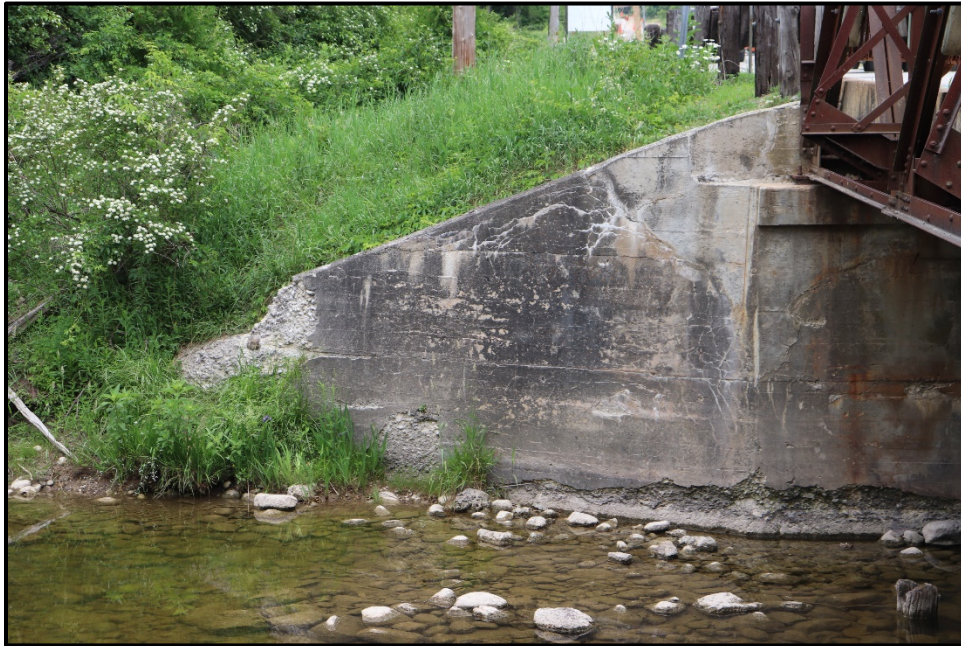
Image 10: Detail of north abutment and east wingwall (TMHC 2020)
