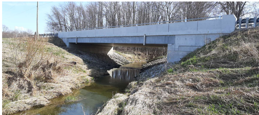
22m span concrete box girders with concrete deck and barrier walls
