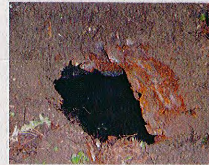
An inspector found this barrel was being used as the septic tank and even the metal lid was corroded.
