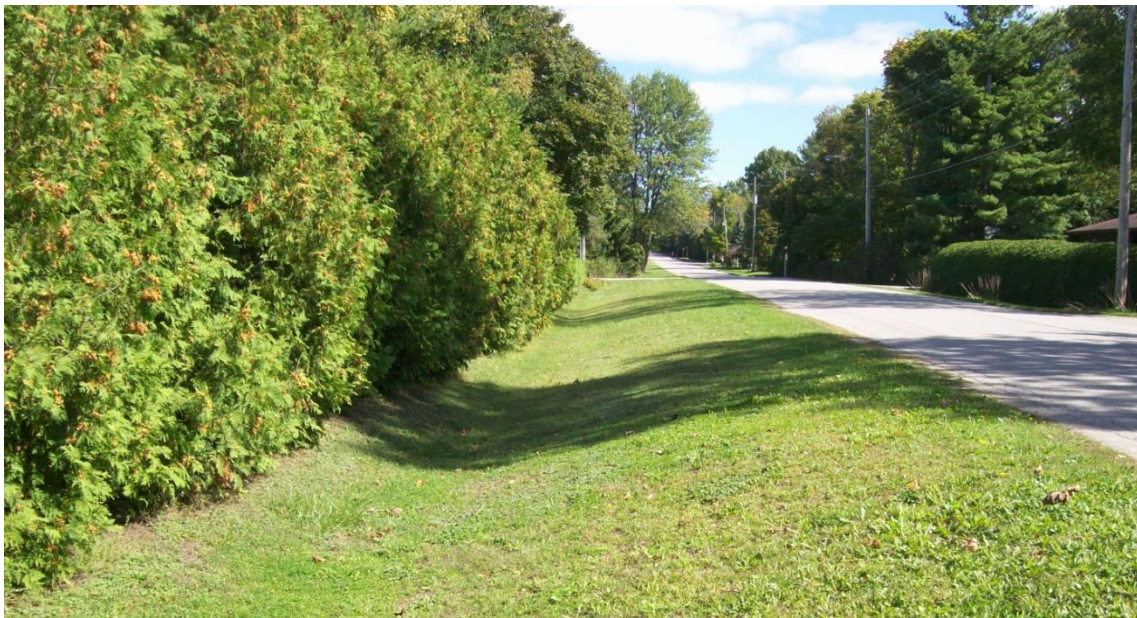
Photo illustrating typical roadside ditch servicing established areas of Bayfield ▲
